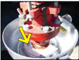
Machined adaptor for fit around the flowline T.
